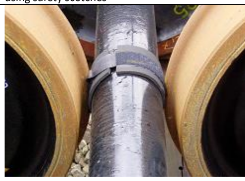
Photo 4: Storing in staggered formation on track with protections against contact
